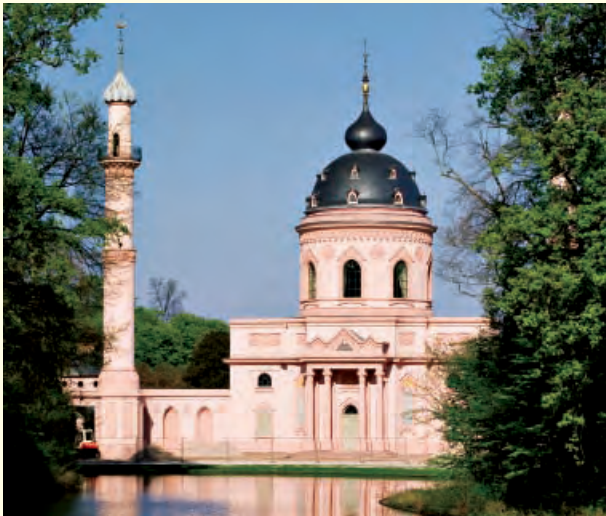
Looking towards the front of the Mosque
